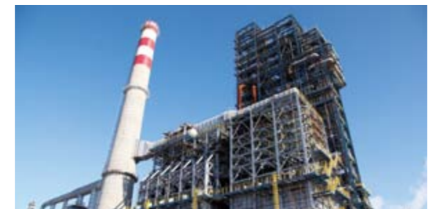
Quanzhou Petrochemical project's continuous reform equipment
