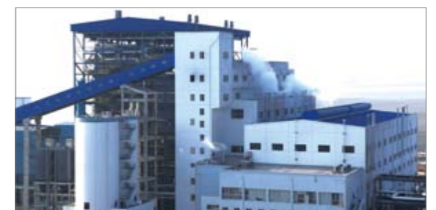
Quanzhou Petrochemical project's power station
